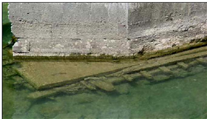
Fig. 7. Round wood foundation base of Konjic Bridge [6]
