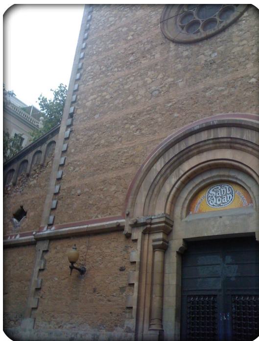
Fig. 14. "banded masonry" in the façade of Saint Joan church in Barcelona
