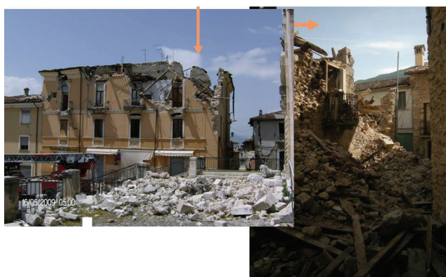
Fig. 3. Problems caused by the irregular and pushing roof timber systems
