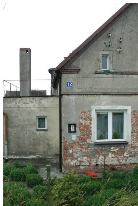
Rys. 6. Monitorowany stary budynek Fig. 6. Monitored old building
