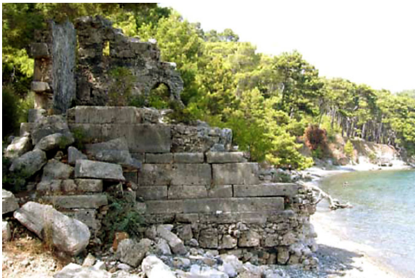
Fig. 5. Foundation of a building in Phaselis Rys. 5. Fundamenty budynku w Phaselis
