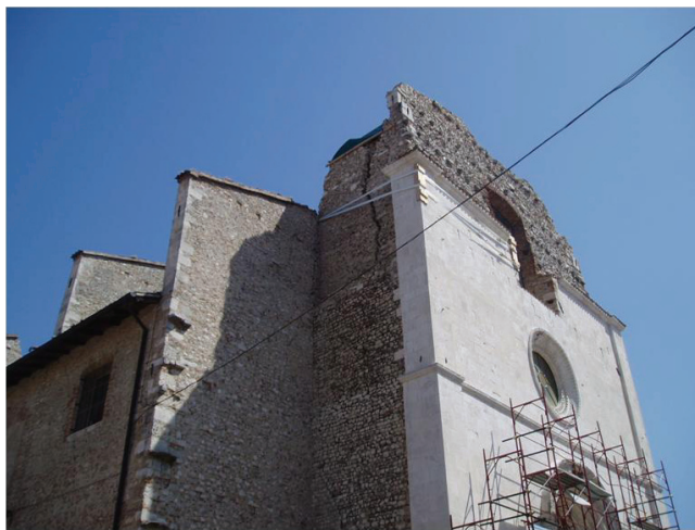
Fig. 13. Slender walls, “two leaves” texture: need to band (Italian: “listare”) it
