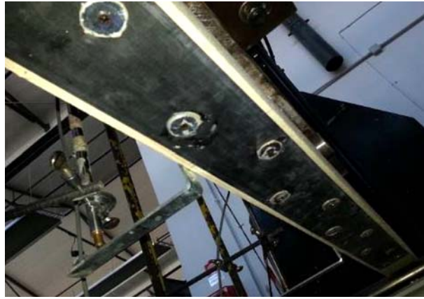
Fig. 5. CFRP plate applied on the timber tension side
