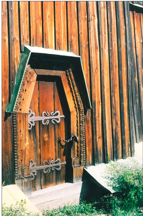
Fig. 6. The carved side jamb of the church; photo by Y. Ivashko.
