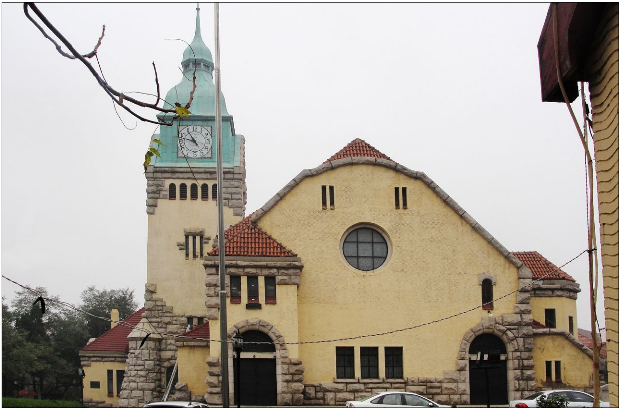
Fig. 5. The south facade of the Protestant Church, present state; photo by Li Shuan.
