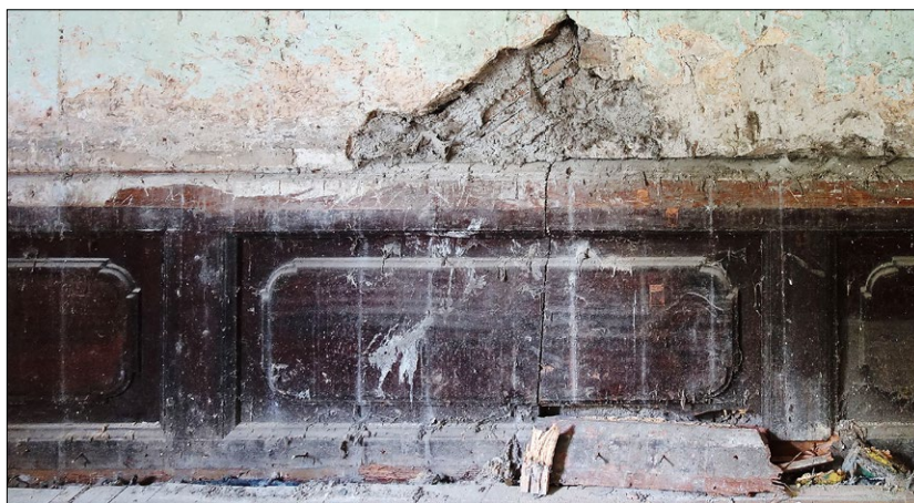
Ryc. 6. Boazeria ścian wewnętrznych pomieszczeń salonu i jadalni; fot. E. Zawaleń 2020. Fig. 6. Wainscoting of the internal walls of the living room and dining room; photo by E. Zawaleń 2020.
