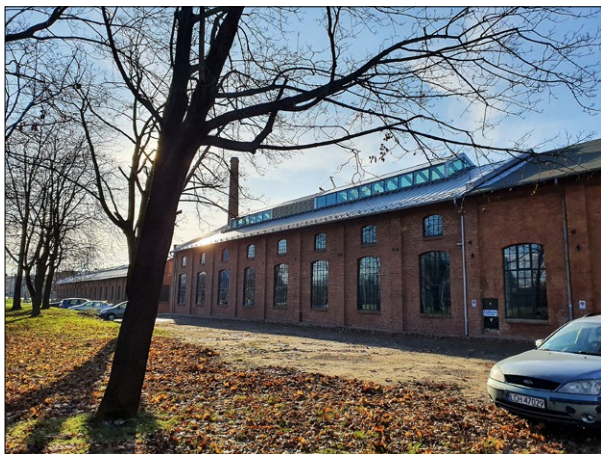
Fig. 1. View of the Petersheim Factory Complex in Cracow – a historical factory complex from the turn of the nineteenth and twentieth centuries, after adaptation and revalorization, 2021; photo by D. Kuśnierz-Krupa
