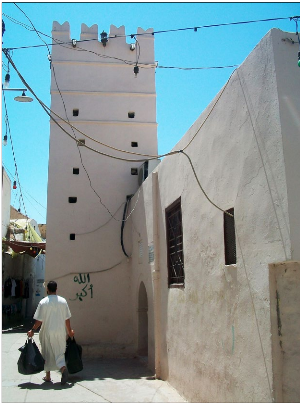
Fig. 3. Al-Naqah Mosque; source: https://upload.wikimedia.org/wikipedia/commons/d/d9/Naga_Mosque_Exterior_Tripoli_Libya.JPG (accessed: 23 XI 2021)
